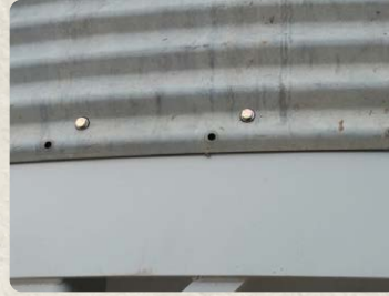
Bolted in valley
