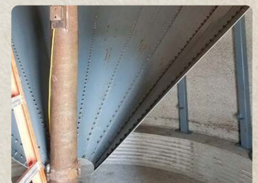
Hopper in Silo
