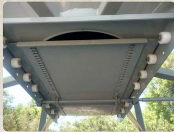
Rack and pinion slide gate
